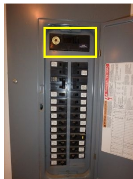
Disconnect in top of panel
