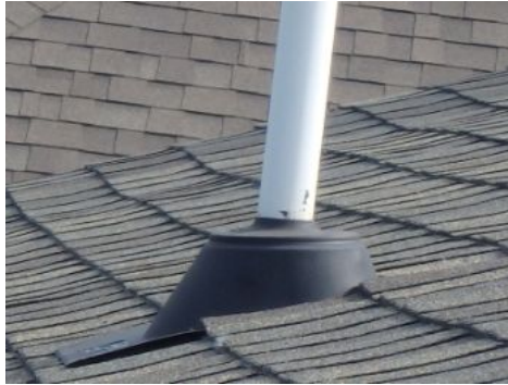
Roof Flashing
