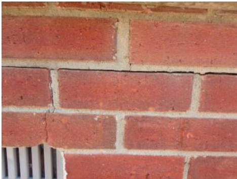
Some settling noted at front porch
