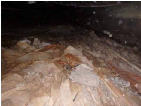
Vapor barrier deteriorated/displaced
