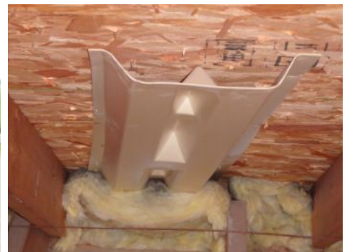
Soffit baffles noted
