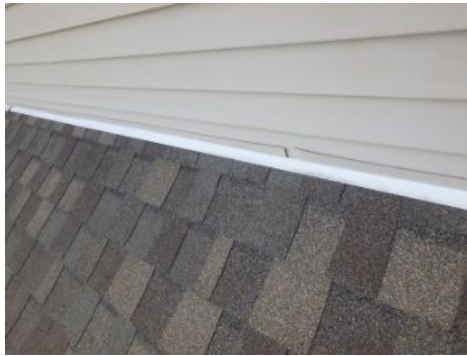
Roof Flashing
