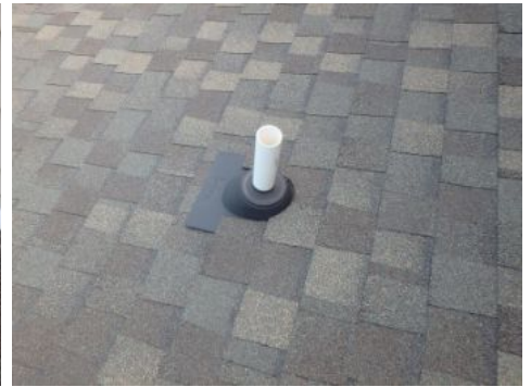
Roof Flashing
