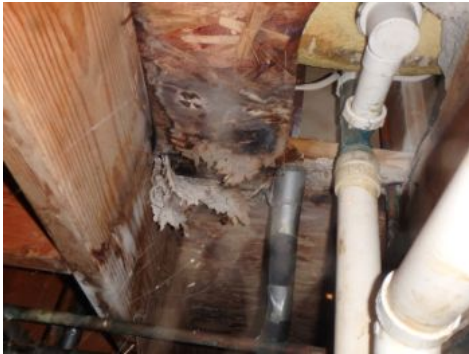
Damaged area under master tub
