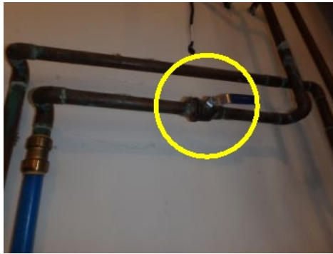
Main shut off above unit
