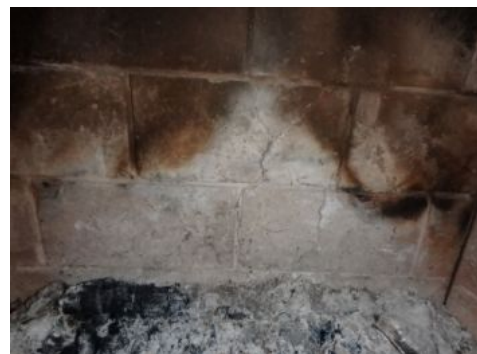
Some cracks noted at refractory panel
