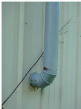
Abandoned HVAC unit vent
