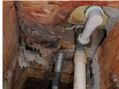
Basement/Crawlspace Subfloor
