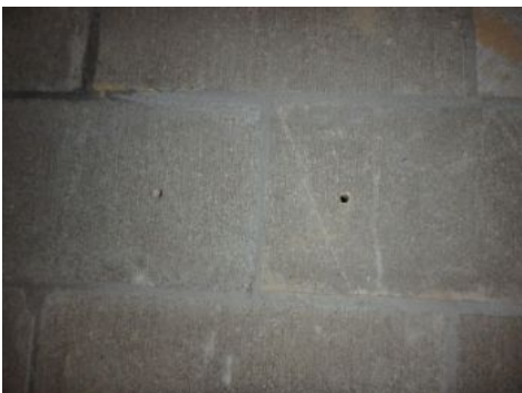
Drill marks from previous termite treatment
