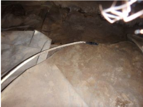
Loose circuit in SE corner
