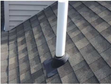
Roof Flashing
