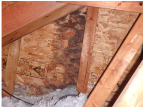
Evidence of past leaks near chimney
